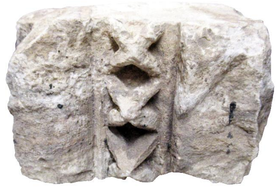
Fig 23. Moulded stone <127> with raised dogtooth ornament between roll mouldings
