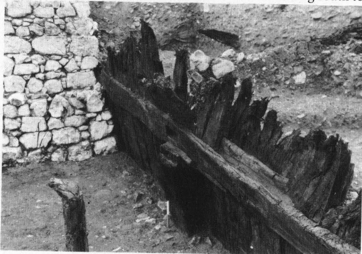
Plate 54. Trig Lane 1974-76: Group 12 revetment second-storey members in west of site. Note groove in upper face of plate; bare-faced tenons on vertical members; repair timbers set behind plate. Looking north-west, river to south, 2×100mm scale.
