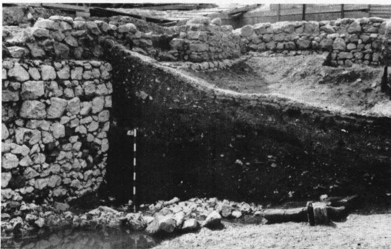
Plate 58. Trig Lane 1974-76: Internal face of Group 15 river wall, looking south-west, river to south. Note exclusive use of ragstone on upper courses; half sectioned dumps sealing chalk rubble raft. 10×100mm scale.
