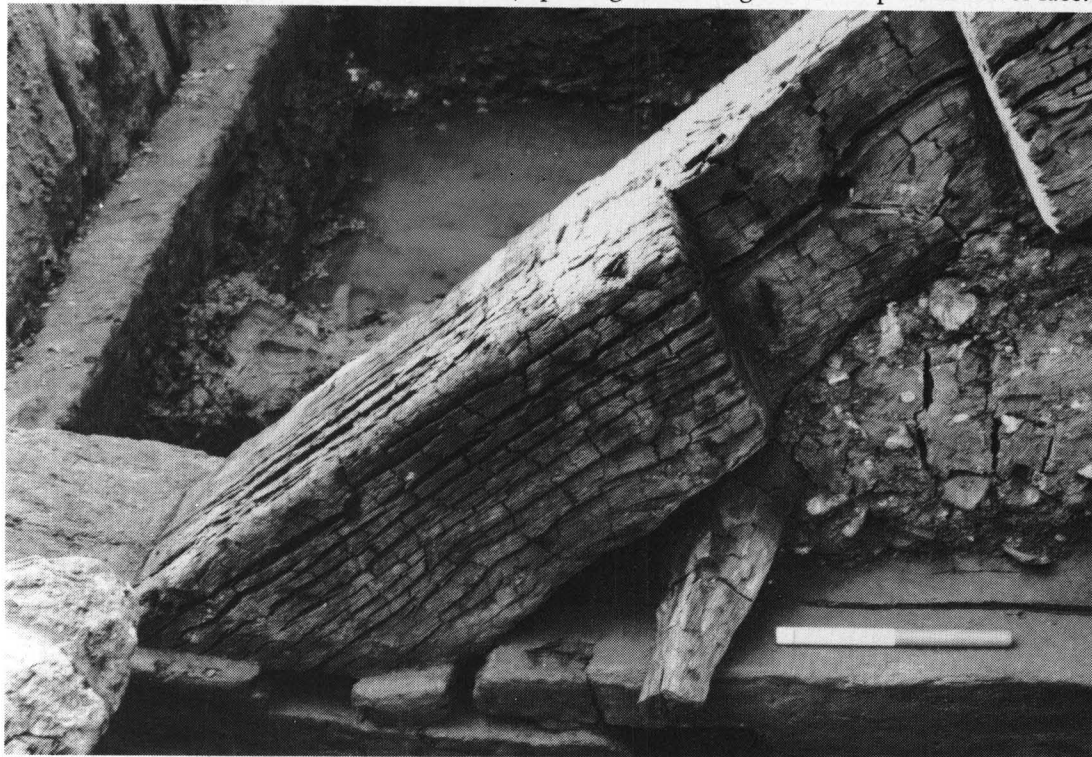
Trig Lane 1974-76: Group 10 back-brace members looking west, showing timbers reused from earlier buildings.
