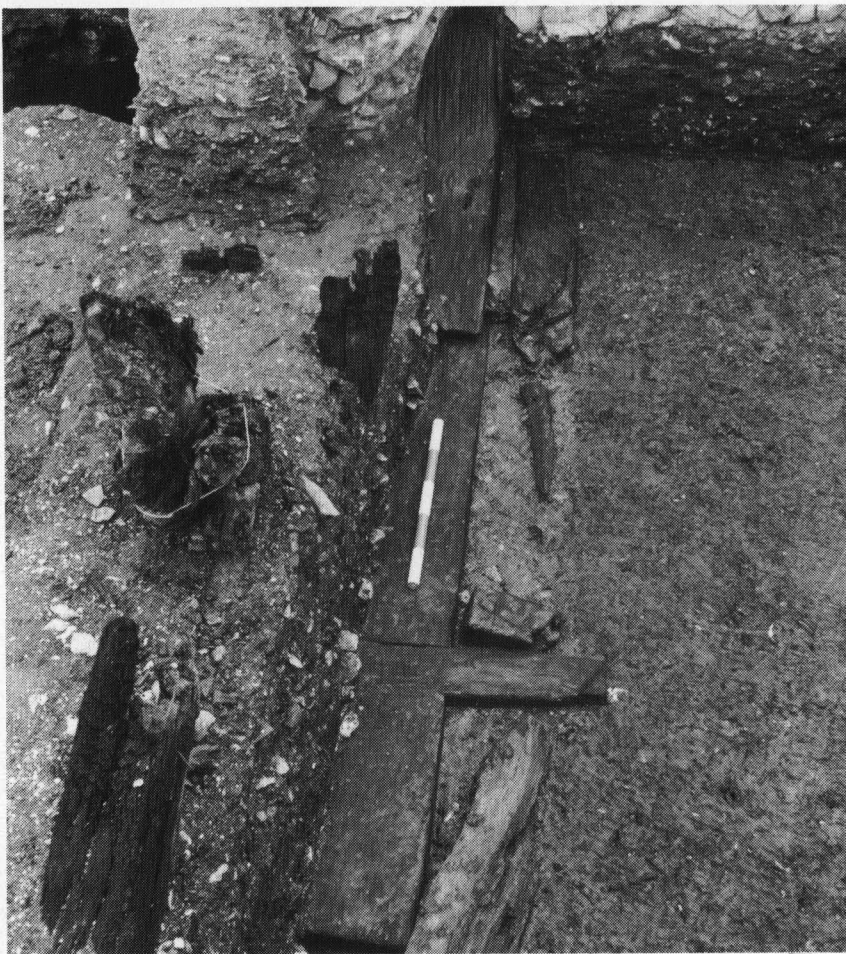
Plate 8. Trig Lane 1974-76: Group 3 revetment back-brace, looking south towards the river. The revetment face lies beyond intrusive stone wall. The cut into which the partially exposed Group 3 tie-back (with 5×100mm scale) was inserted is clearly visible, packed with timber fragments derived from earlier Group 1 structure B to east.
