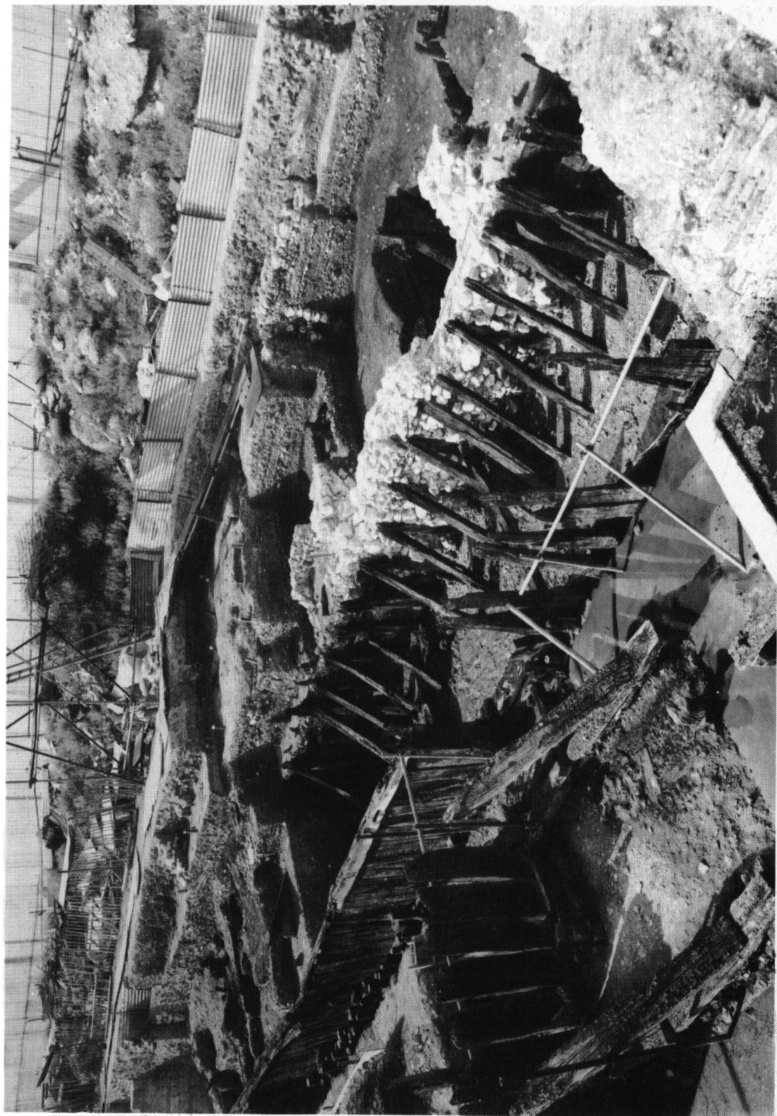
Plate 4. Trig Lane 1974-76: Front-braced Group 3 revetment cut by later chalk foundation, looking north-west, river to south. The subsidiary base-plates are buried beneath the foreshore which accumulated against the revetment's southern face. 4x500mm scale.
