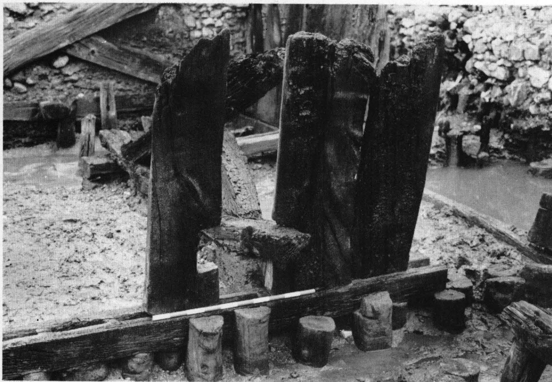
Plate 49. Group 11 revetment. Utilising the double-length mortise, the 3rd vertical member trenched on its southern edge, is slid into position. Looking south-east. 10×100mm scale.
