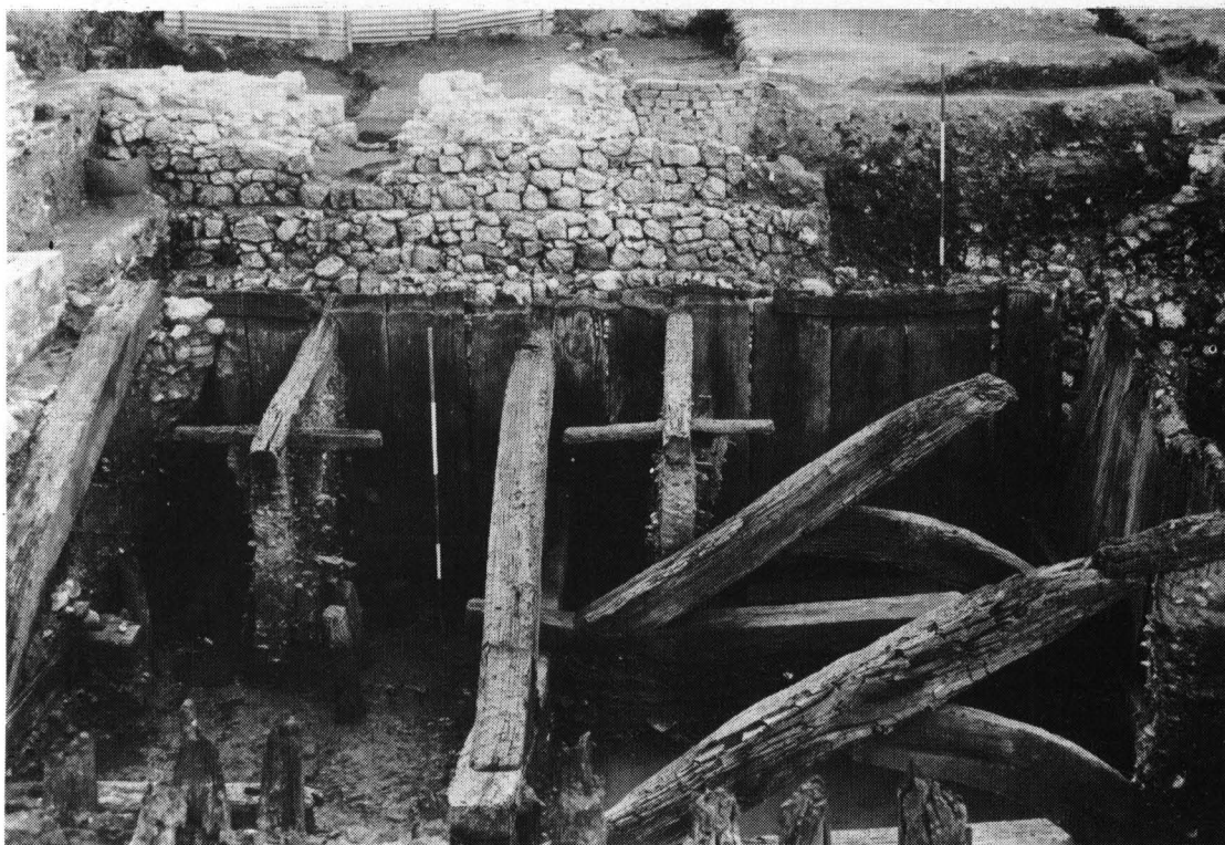
Plate 41. Trig Lane 1974-76: Internal face of Group 11 revetment's southern wall, looking south towards the river. 4×500mm scale.
