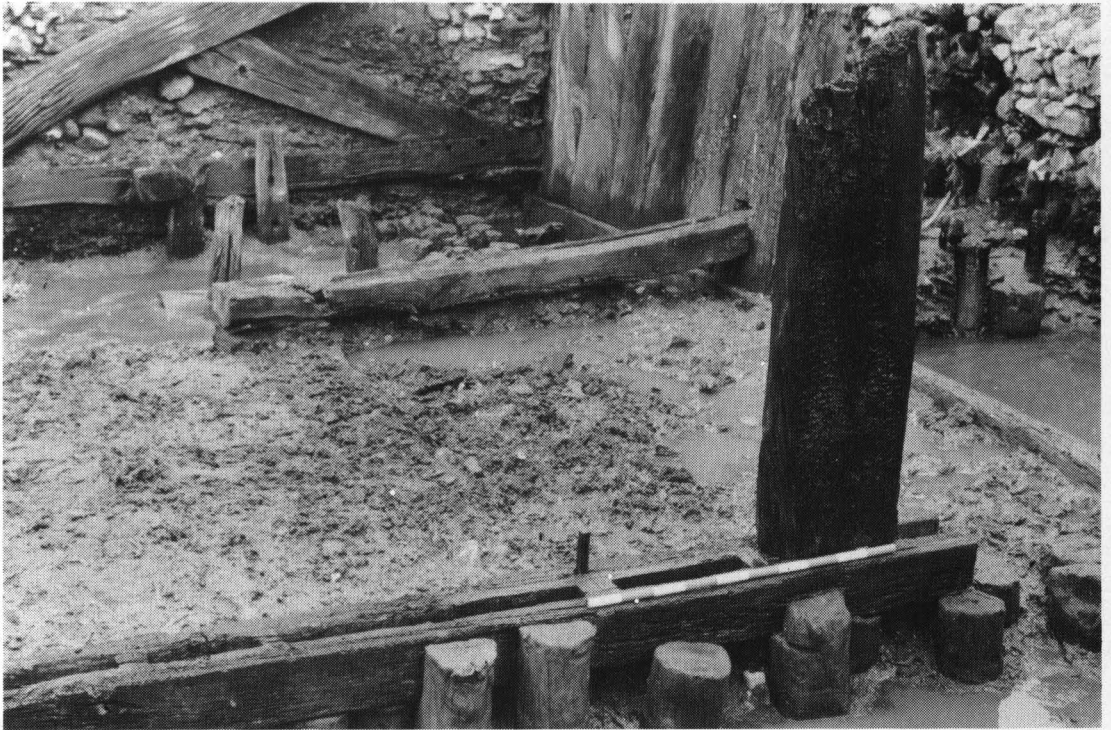
Plate 46. Group 11 revetment. First vertical member in situ , looking south-east. 10×100mm scale.
