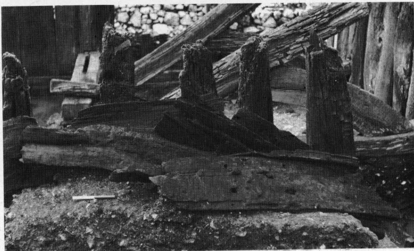
Plate 20. Trig Lane 1974-76: Internal face of Group 7 revetment showing rivetted overlapping strakes from clinker-built boat reused as cladding. Looking south towards river, 2×100mm scale.
