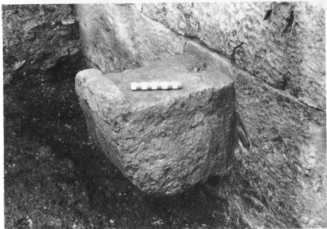
Plate 62. Trig Lane 1974–76: Corbel from Group 15 river wall which supported timber stair to foreshore. Note (?) bolt to north of 10×10mm scale. Looking west, river to south.
