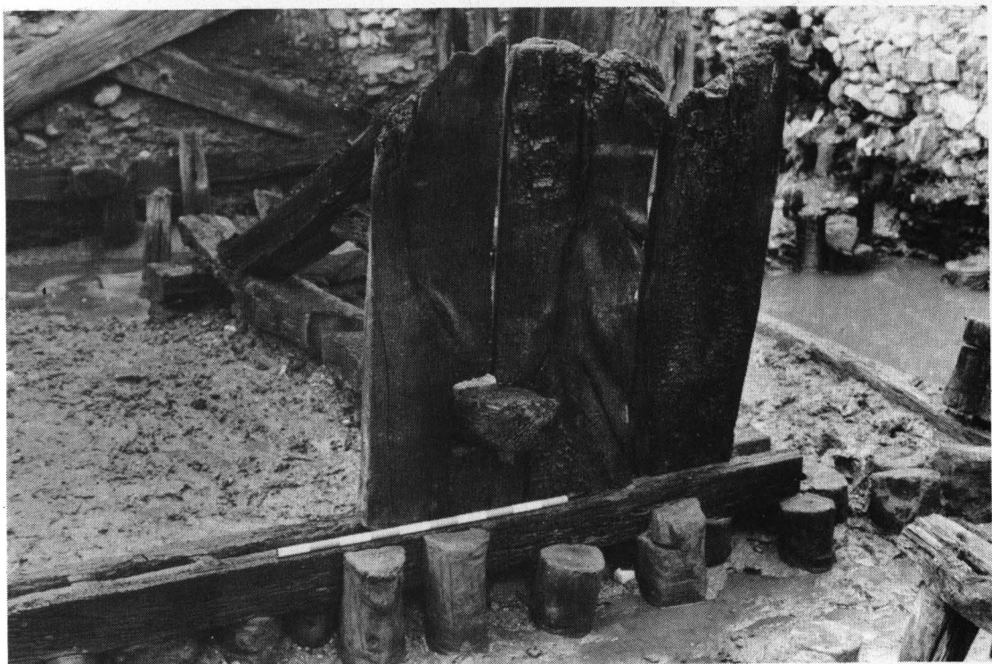
Plate 50. Group 11 revetment. 3rd vertical member in position. Looking south-east. 10×100mm scale.
