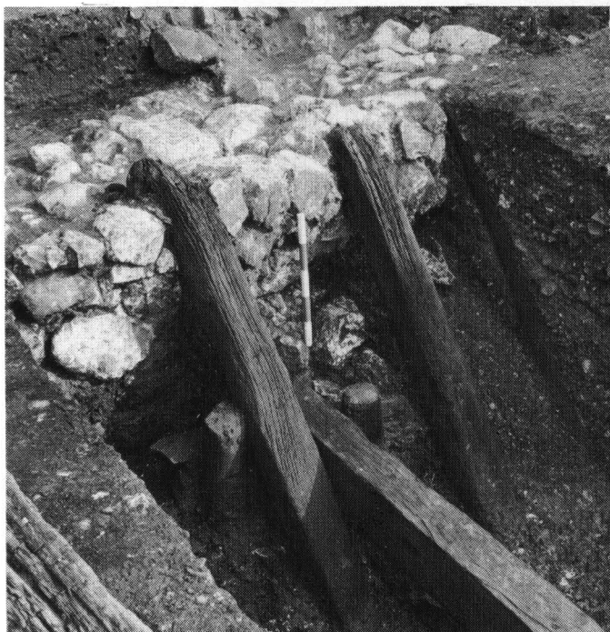
Plate 18. Trig Lane 1974–76: Group 7 revetment tie-back, cross-piece and earlier Group 3 revetment front braces partially encased in the stone foundation. Looking north-east, river to south, 5×100mm scale.
