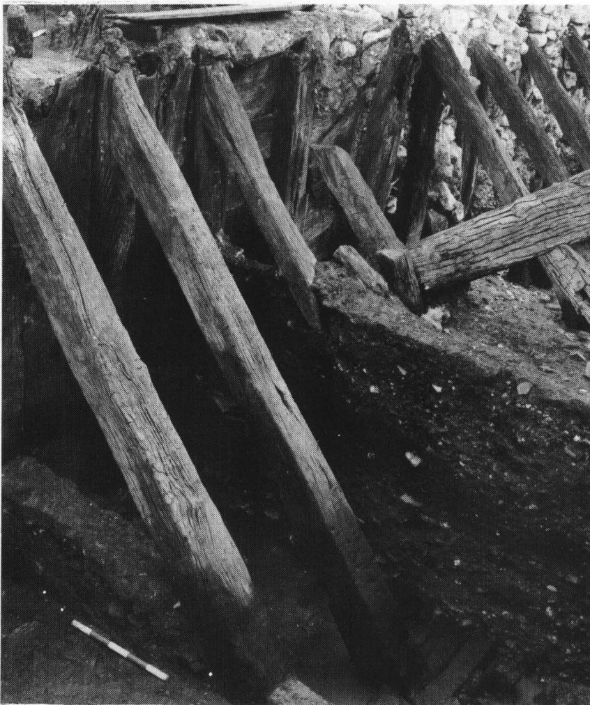
Plate 6. Trig Lane 1974-76: Group 3 revetment face showing 2.5m long diagonal brace running from head of post to subsidiary base-plate. Looking north-east, river to south, 5×100mm scale.
