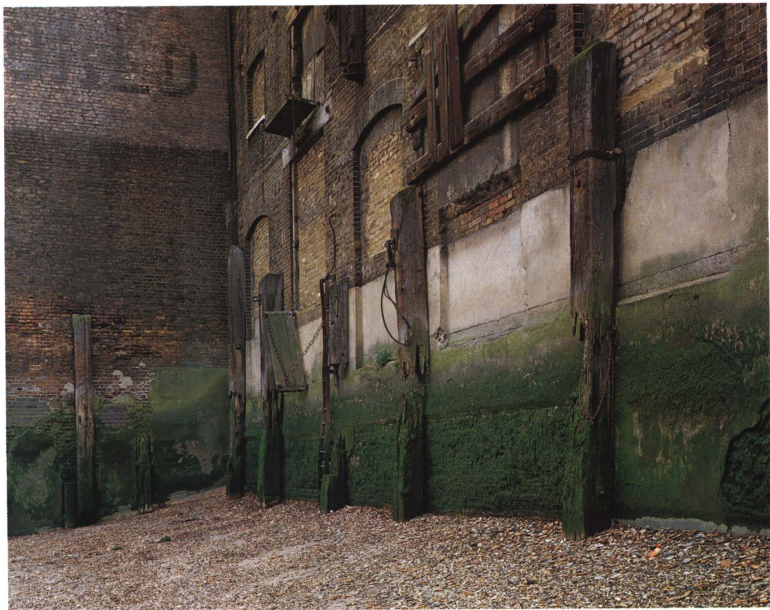
Plate 72. Trig Lane 1974-76: Rubbing posts decaying on the line of the Mean High Water Neap tides on present day Thames Foreshore. The timber above and below this level is sound. Note position of scarf joints.
