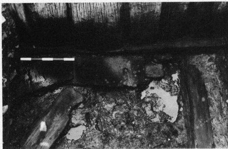
Plate 30. Trig Lane 1974-76: Planking presumably derived from the Group 7 revetment (with 5×100mm scale) reused as walk boards facilitating the construction of the Group 10 revetment, the internal face of which is visible at top of picture. Looking south.
