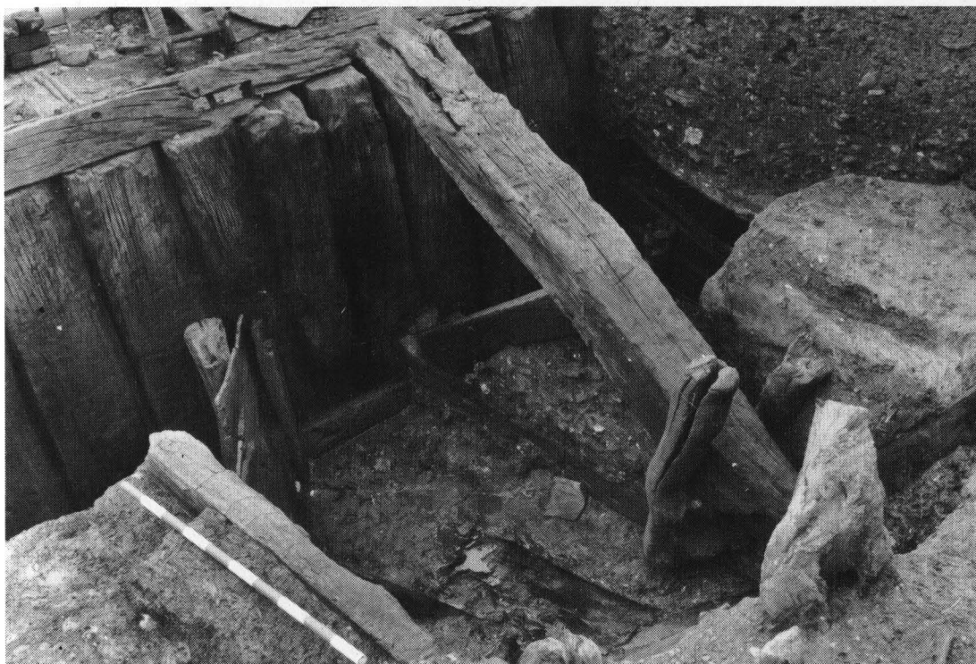
Plate 25. Trig Lane 1974–76: Group 10 revetment Brace 4, looking south-west towards river. The stave-built revetment replaced the Group 7 revetment. Right of the 10×100mm scale is a Group 7 tie-back in situ severed at its southern end by cut which removed its associated revetment. To its right is 2m wide cut through the Group 7 dumps in which Group 10 brace was erected. Note shuttering to east & west of brace enclosing an area which had to be backfilled before construction work could progress eastwards.
