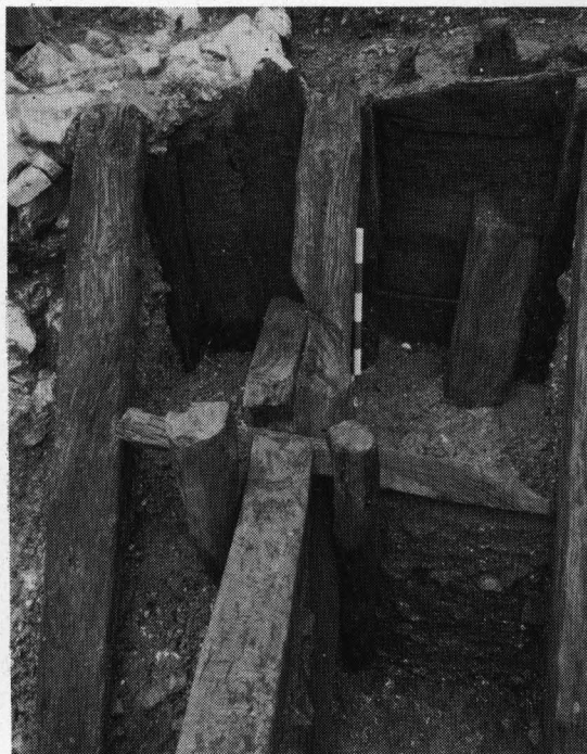
Plate 19. Trig Lane 1974–76: Group 3 revetment brace cut to accommodate later Group 7 revetment tie-back and pile retained cross-piece. Axe marks clearly visible to right of 5×100mm scale. Northern end of tie-back broken off. Looking north, river to south.
