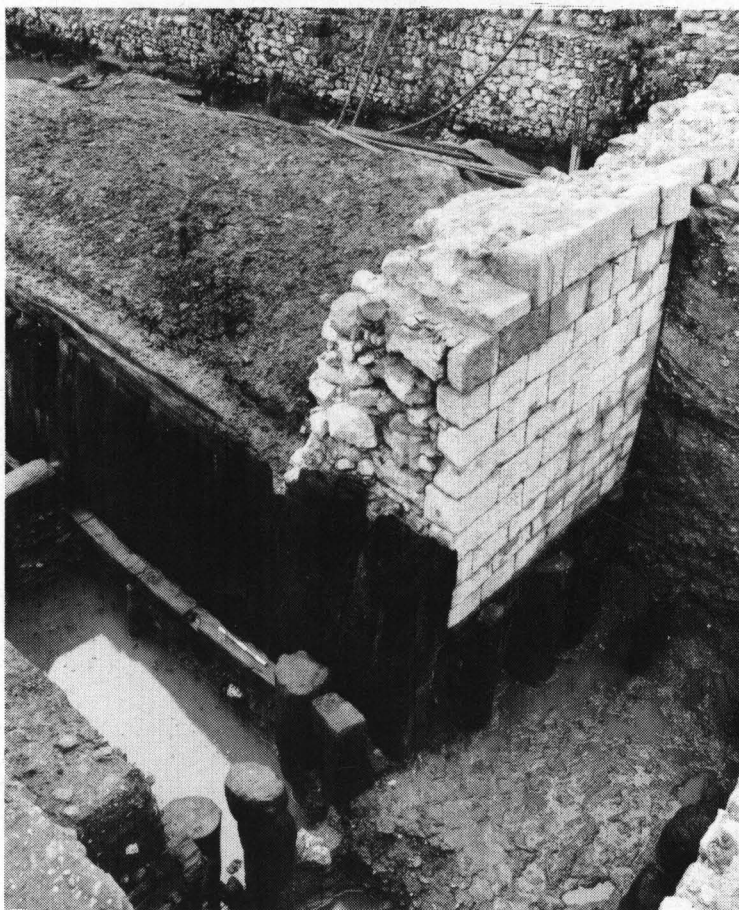
Plate 59. Trig Lane 1974-76: Dressed ragstone on external face of Group 15 river wall, looking south-east, river to west. The wall is built on foreshore which accumulated against Group 10 revetment, with 5×100mm scale.
