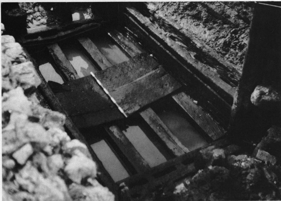
Plate 38. Trig Lane 1974-76: Platform feature on south-west corner of Group 11 revetment, looking north-west, with planking removed to reveal joists. Note mortises in frame members for a tank-like superstructure, and revetment stave on right tenoned into platform frame. 10×100mm scale.
