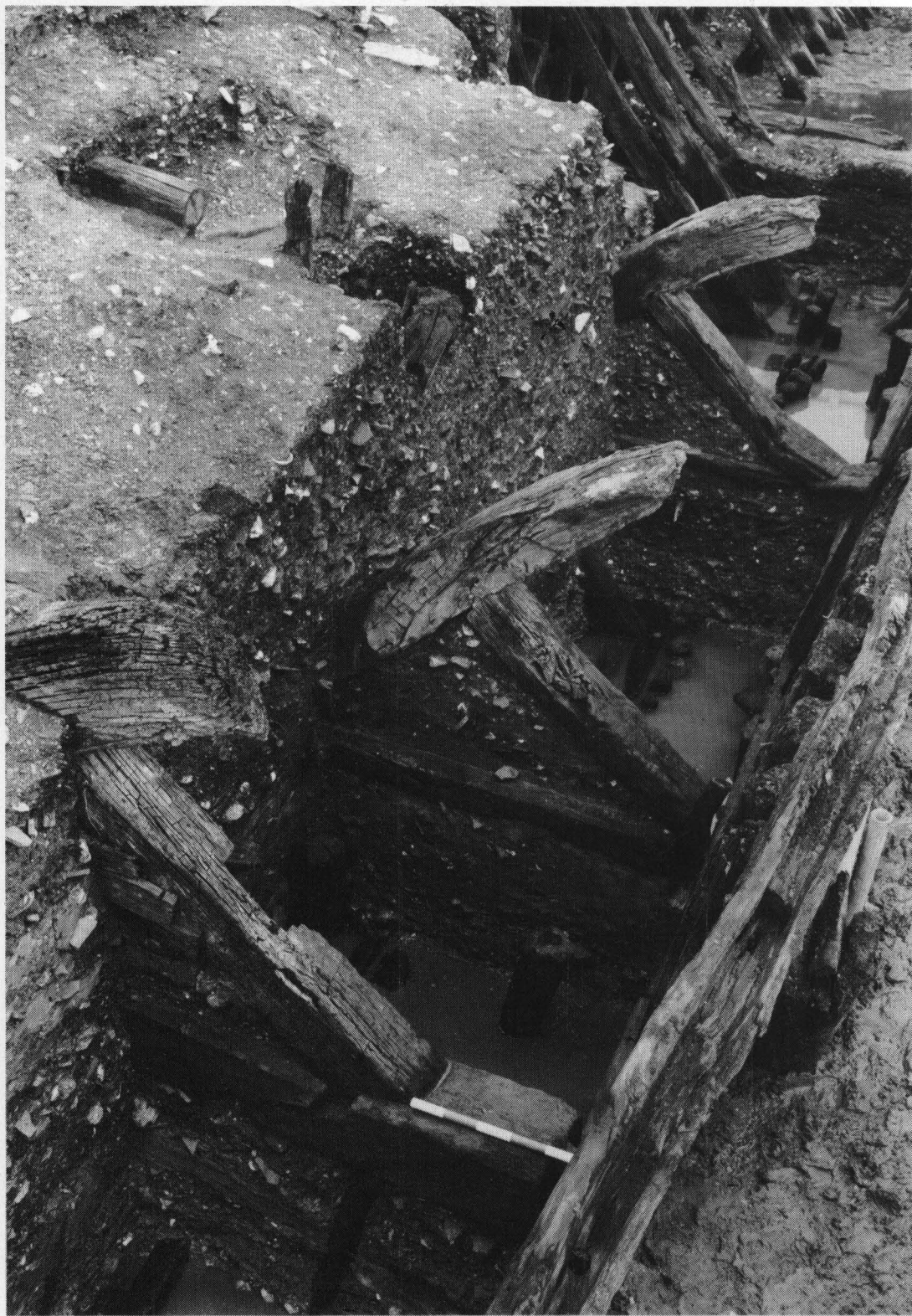
Plate 23. Trig Lane 1974-76: Group 10 back-braces laid on dumped deposits overlying foreshore sealing earlier Group 3 & 4 subsidiary base-plates. Looking north-east, river to south, 5×100mm scale.
