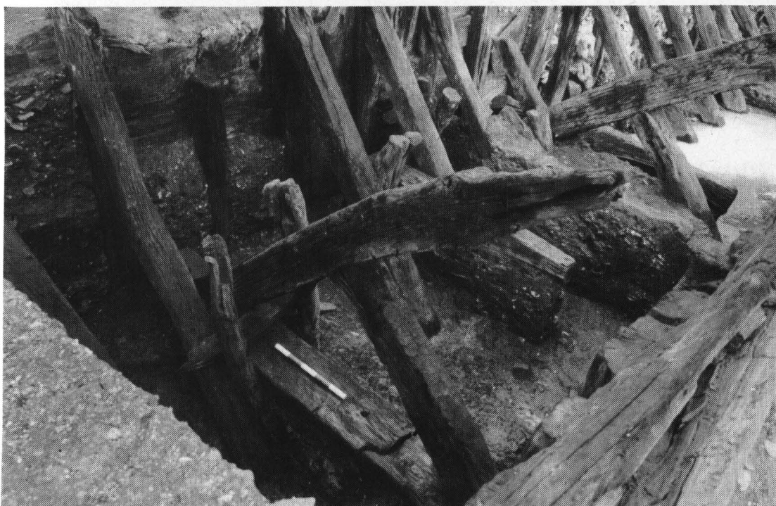
Plate 24. Trig Lane 1974–76: Group 10 revetment back-brace with 5×100mm scale supported by piles and cross-piece wedged against earlier Group 3 brace. Group 7 tie-back to east with southern end severed when associated revetment face replaced by stave wall to right. Looking north-east, river to south.
