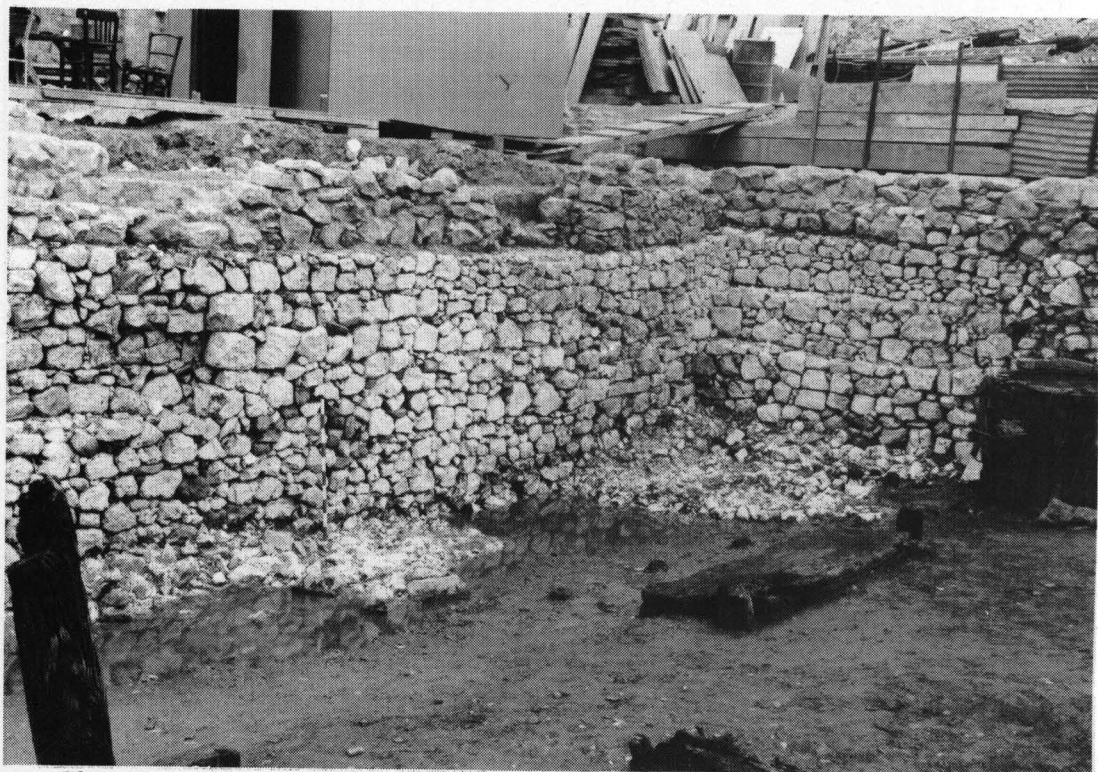
Plate 56. Trig Lane 1974-76: Internal face of Group 15 wall, showing construction of south-west corner. Looking south-west. 10×100mm scale.
