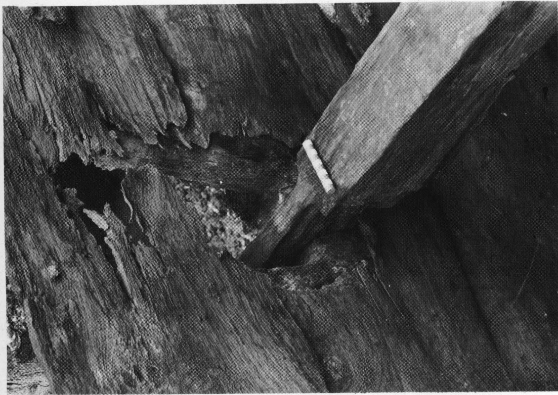
Plate 16. Trig Lane 1974-76: Group 7 tie-back pushed through crudely made hole in revetment planking. Looking south-west, river to south, 10x10mm scale.
