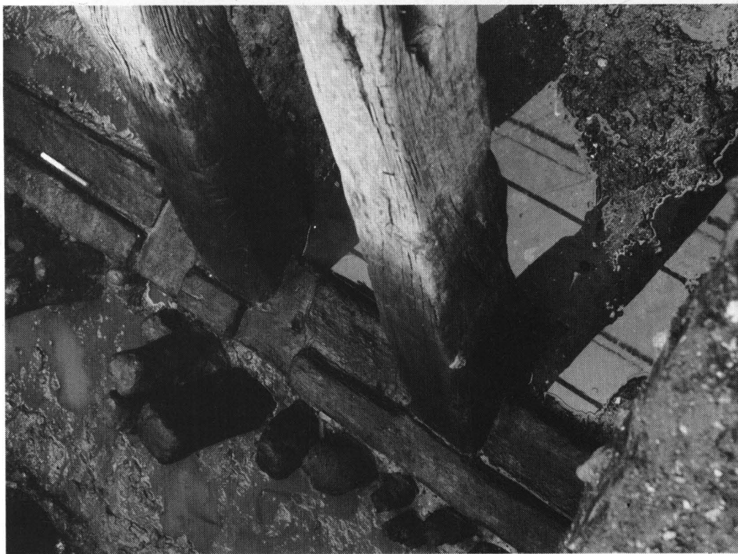
Plate 7, a and b. Trig Lane 1974-76: Group 3 subsidiary base-plate with 2x100mm scale looking east, river to south. Note retaining piles and bird's-mouth abutment at foot of braces, a joint which is neither tenoned nor pegged. Traces of dove-tail joint on base-plate show it was reused.
