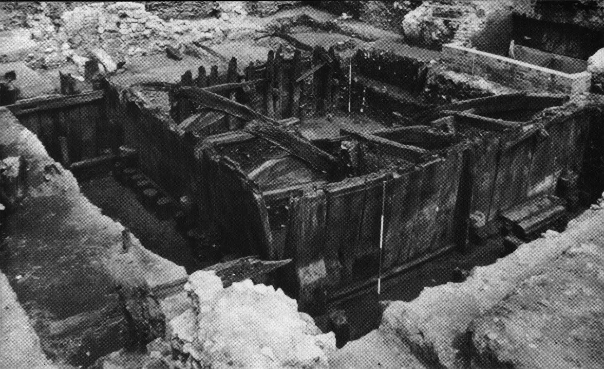
Plates 36 and 37. Trig Lane 1974–76: South and west walls of stave-built Group 11 revetment with infill material removed. River to south and west, 4×500mm scales. a) looking north b) looking north-east.
