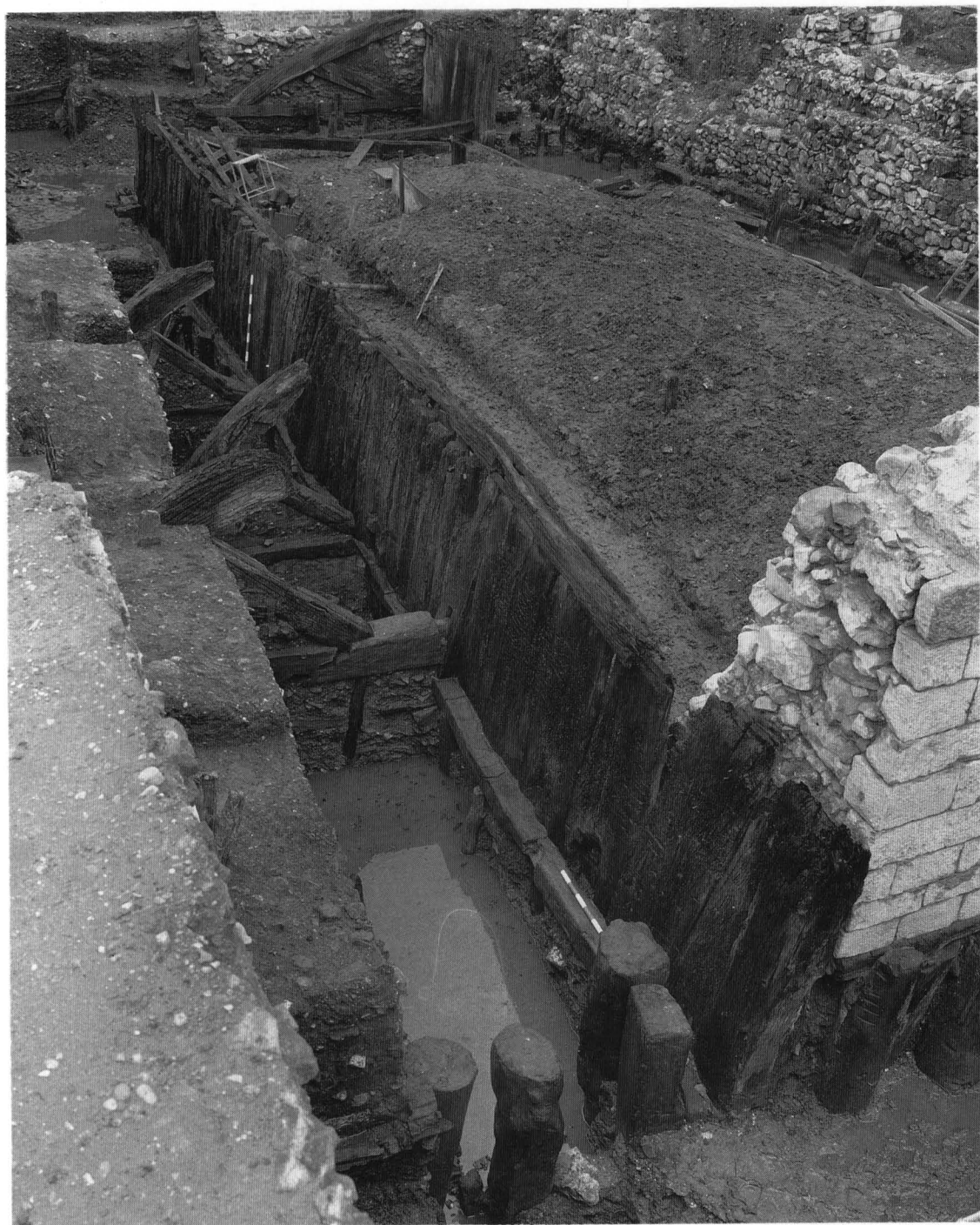
76. Trig Lane: north (landward) face of TL10 revetment, looking east. The horizontal 5 x 100mm scale rests on the grooved baseplate into which the staves were set: three triangular back braces which supported the 16m-long stave wall from behind have been partially exposed in the trench cut through the infill deposits.
