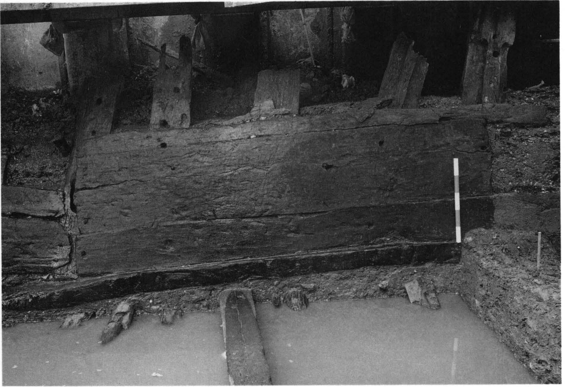
25. Billingsgate Lorry Park: landward (north) face of BG16 revetment excavated on the edge of the sheet-piled southern limit of excavation. The 5 x 100mm scale stands on baseplate into which posts were set. Note rebates on two posts in west (right), showing that they were reused timbers (cf. Fig 24).
