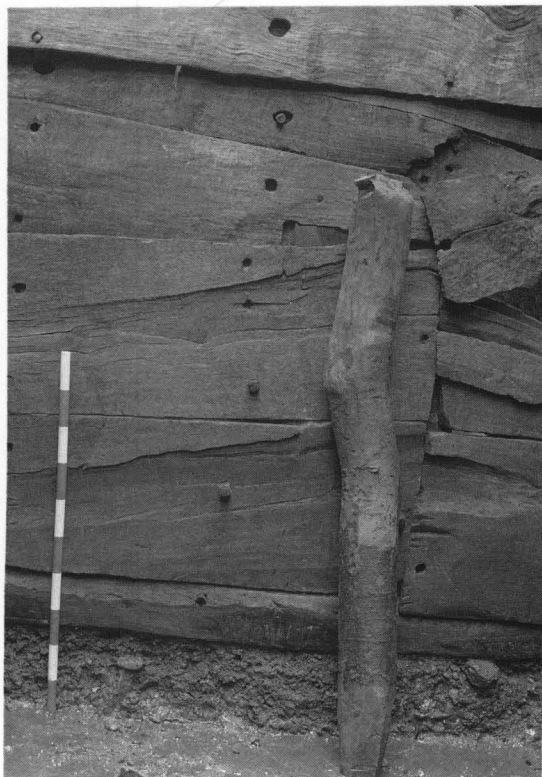
36. Seal House: landward face of SH4 revetment, looking south. The 10 x 100mm scale rests against the plank cladding which has been pegged to the revetment posts.
