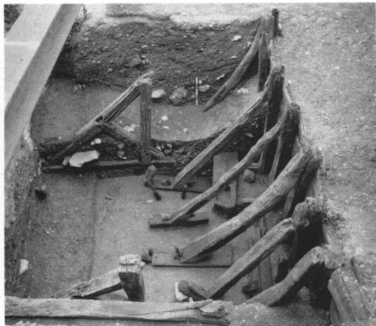
54. Thames Exchange: part of the 13th-century waterfront, looking east. The 5 x 100mm scale stands on the foreshore which accumulated against the face of the TX4 revetment, to right, surviving almost to full height. In centre of area, a trench has been cut down to the base of the TX5 jetty trestle, erected in the open river to the south of the revetment.
