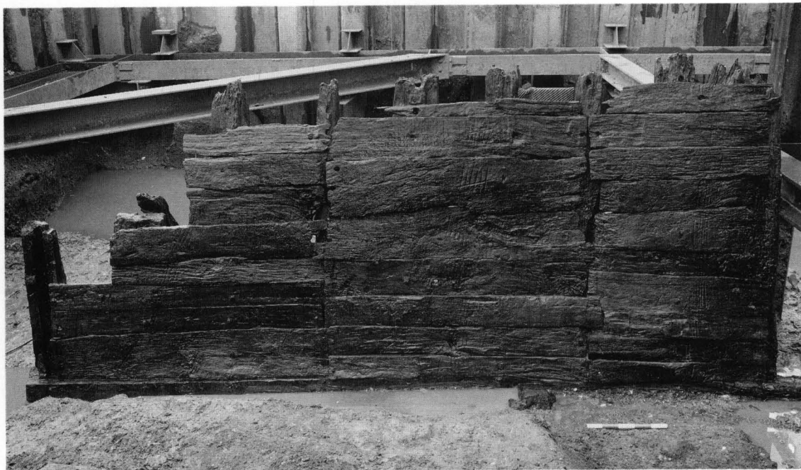
23. Below: Billingsgate Lorry Park. BG14 revetment cladding as on Fig 22, but with the assembly marks enhanced with chalk.
