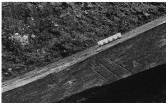
52. Thames Exchange: detail of TX4 revetment back brace, looking east. The 10 x 10mm scale rests on a squared timber above an incised assembly mark (cf. Fig 51c).
