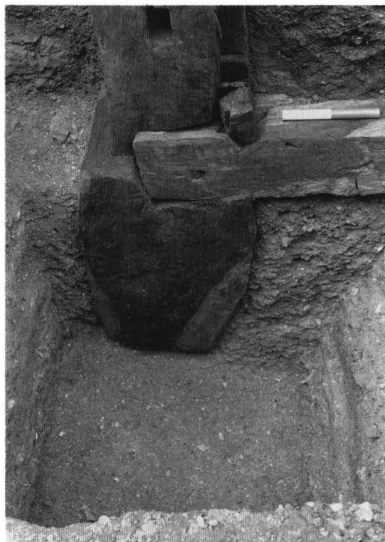
84. Thames Exchange: detail of early 13th-century TX4 revetment, showing the base of an earthfast post exposed in a trench cut through the foreshore deposits. The 2 x 100mm scale rests on a back brace which is joined to the post with a pegged notched lap joint.
