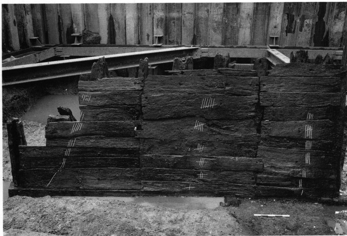
22. Above: Billingsgate Lorry Park. Reverse (landward) face of BG14 revetment cladding, looking south. The unenhanced assembly marks (cf. Fig 23) show that it was prefabricated; scale 5 x 100mm.
