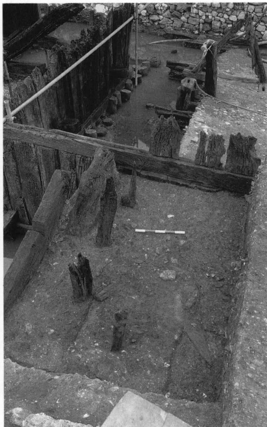
81. Trig Lane: general view of part of the bipartite TL10/G12 revetment, looking south. The 5 x 100mm scale rests on an excavated horizon within infill deposits dumped to north of (behind) the stave-built 14th-century TL10 revetment. Over the top of the stave wall sits a grooved baseplate, part of the 15th-century G12 revetment, into which a line of vertical planks were set, of which the remains of three can be seen.
