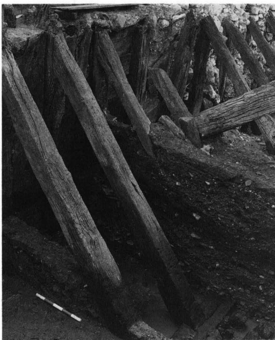
70. Above: Trig Lane. Two squared front braces from TL3 revetment, looking north-east. The 5 x 100mm scale rests on the foreshore upon which the principal baseplate was laid, just visible to left (north). Note the bird's-mouth abutment on the foot of the brace, where it meets the partially-exposed subsidiary baseplate.
